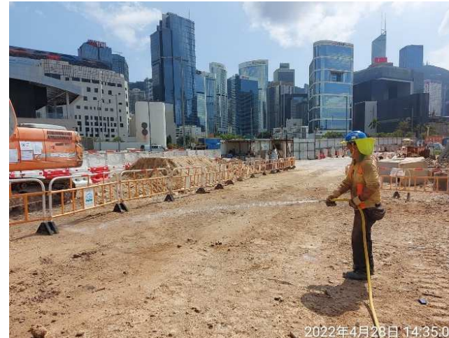
定期灑水抑塵 Regular water spraying for dust suppression
