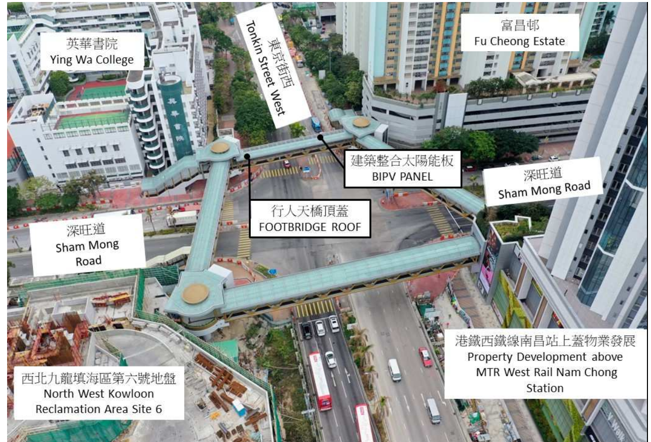
已裝設整合太陽能板的深旺道行人天橋系統 Sham Wong Road Footbridge System with Installed BIPV Panel
