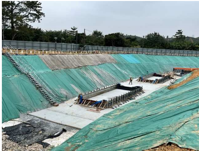
以帆布幅蓋挖掘面 Covering excavated surface by tarpaulin sheet
